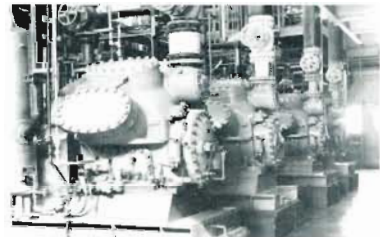
150 Ton Ammonia Compressor in the Foreground
